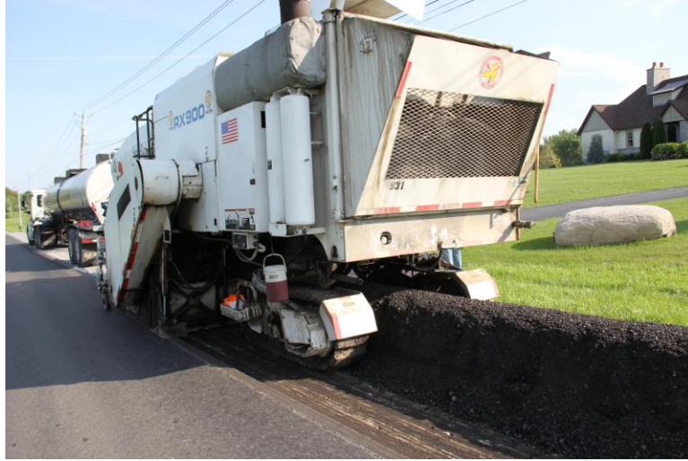
Figure 4. CIR Mix Placement (Suit-Kote, 2019)
