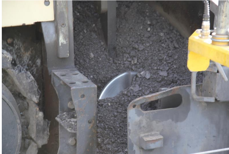
Figure 3. CIR Mixing Process (Suit-Kote, 2019)
